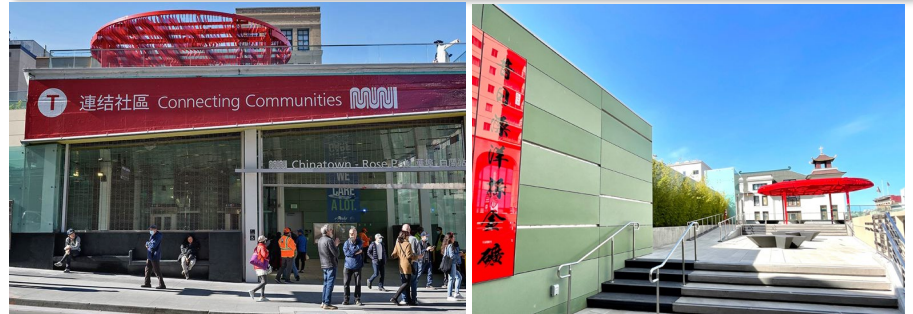
SF Central Subway Chinatown-Rose Pak Station
