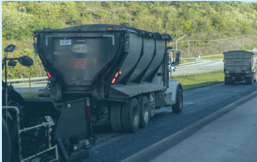
Project truck hauling
