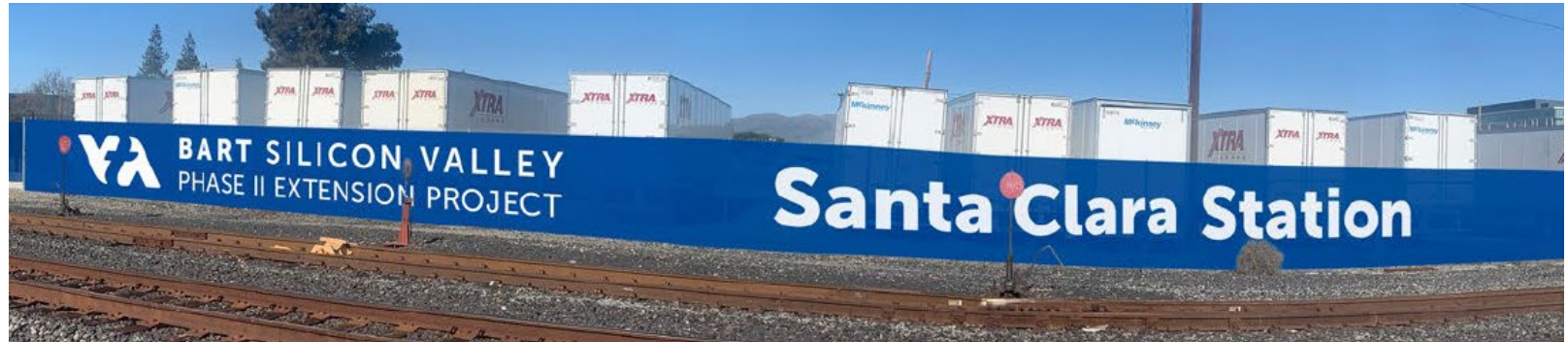
Potential screening on Project fences at Santa Clara station – Subject to Change
