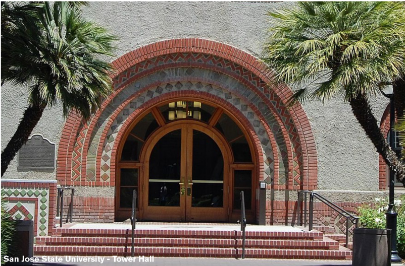
San Jose State University - Tower Hall
