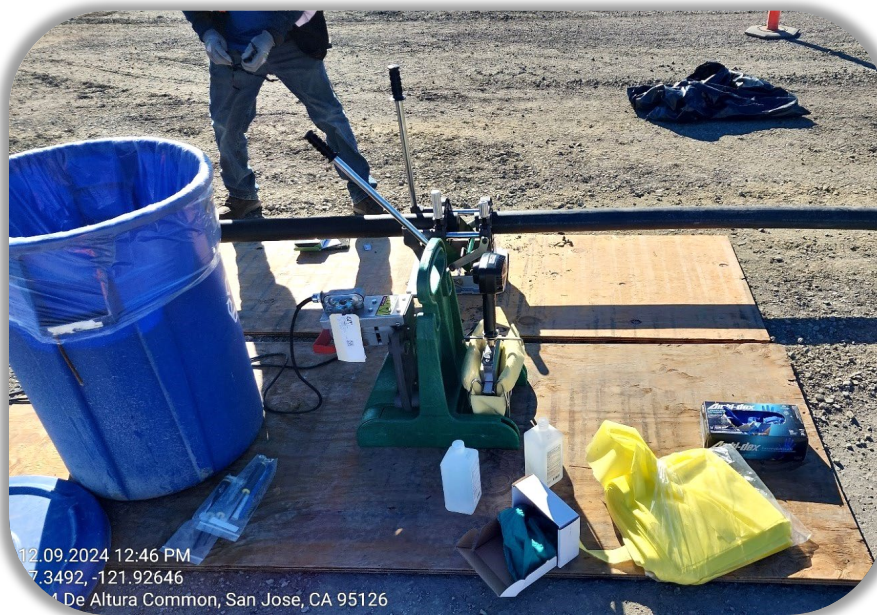
Fusing HDPE Air Line Prior to Installation
