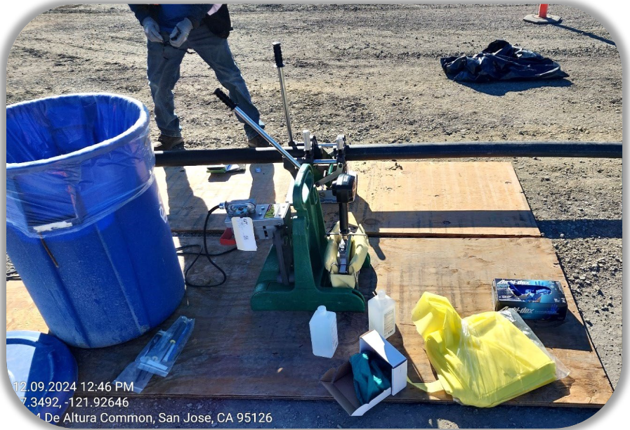
Fusing HDPE Air Line Prior to Installation
