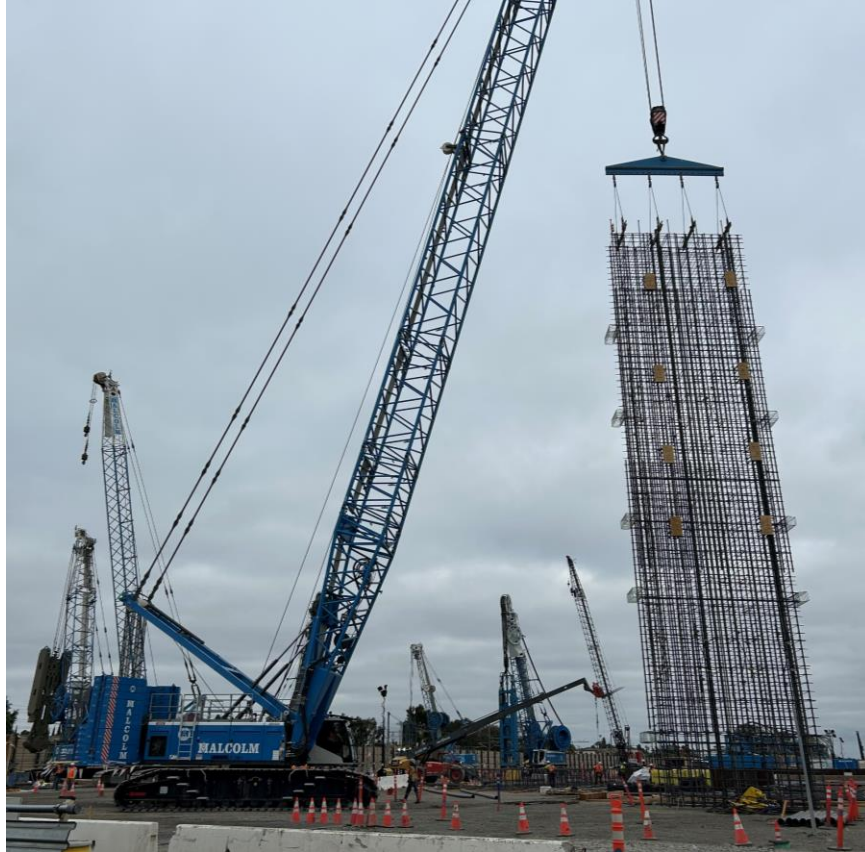
Rebar cage being lifted for underground support wall construction.
