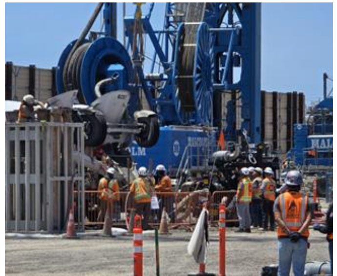
Underground support wall concrete being poured.
