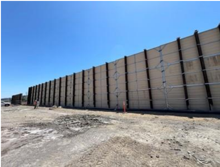
Completed soundwall framing and panels.
