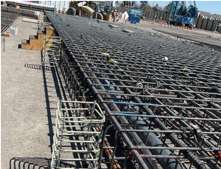
Rebar cage prior to lift and installation.
