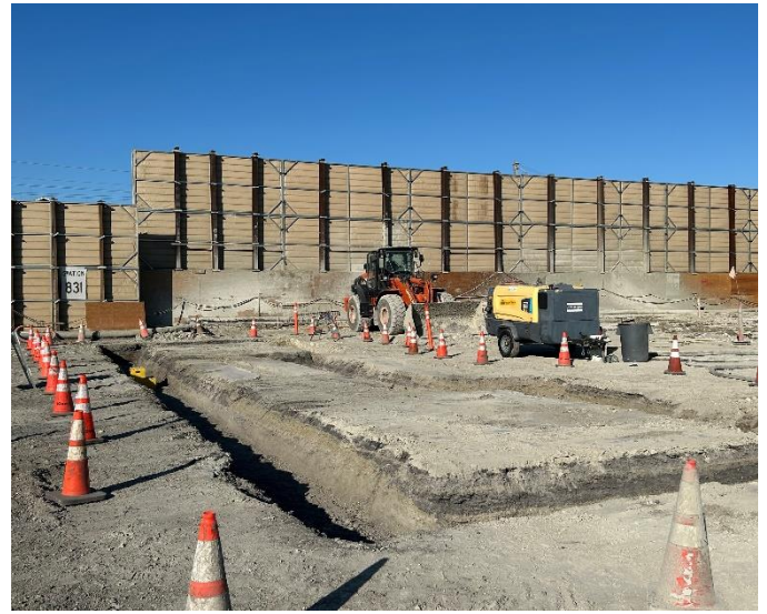
Excavation of guide wall for ground improvements.
