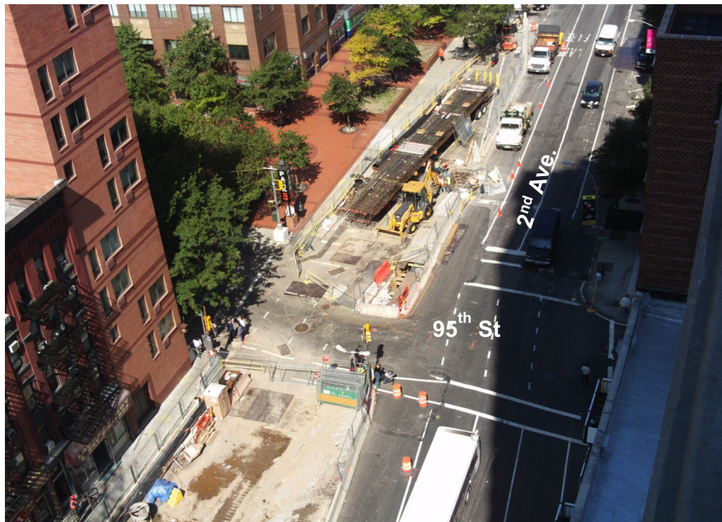
Figure 14 – Staged Construction Across a Side Street - Second Ave. Subway - NY
