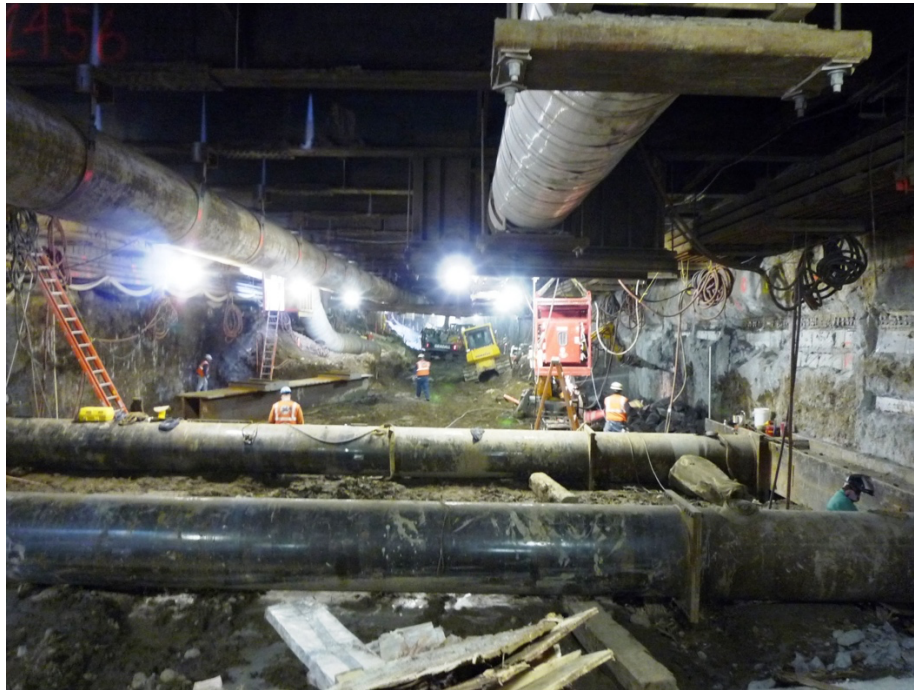
Figure 15 – Decking Beams and Support of Utilities - Second Ave. Subway - NY
