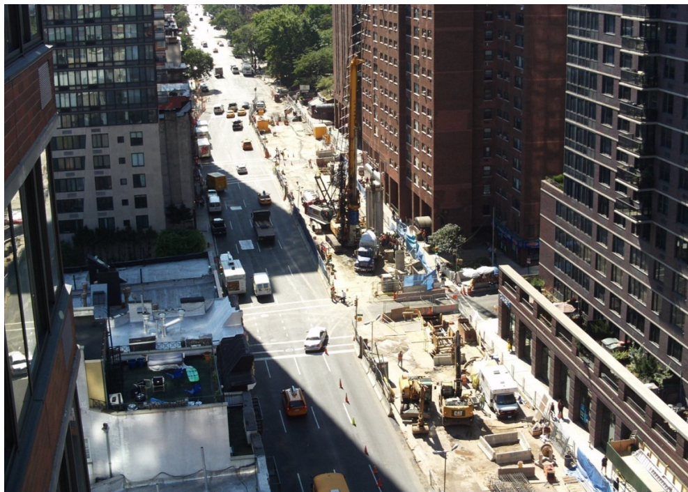
Figure 12 – Slurry Wall Installation – Typical Work Zone - Second Ave. Subway - NY
