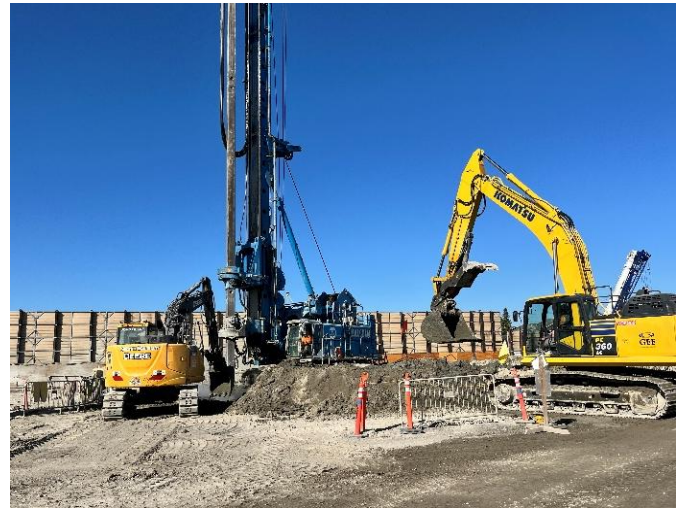
Heavy equipment being used to excavate and remove soil where ground improvements are being made for greater stability of the launch structure.
