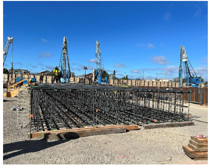
Assembling a large rebar cage that will form the underground launch structure walls.
