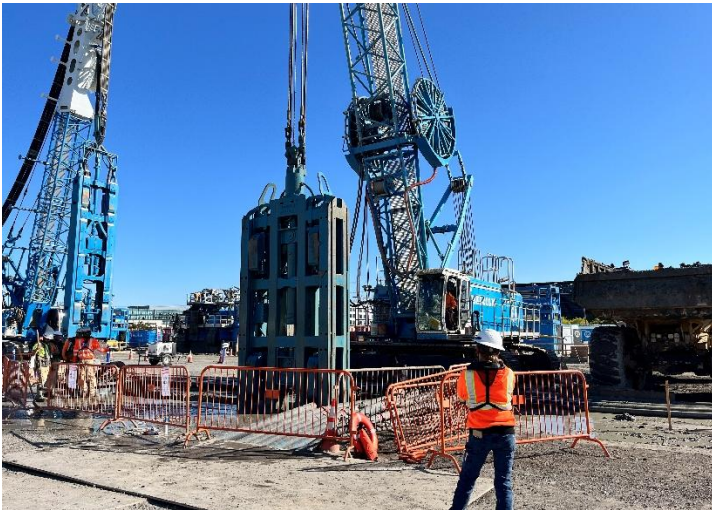
The crane excavating soil to support guidewall construction for the launch structure.
