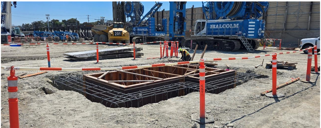
Formwork and rebar installation completed for foundation elements at West Portal. This work supports the upcoming caterpillar shaft construction.
