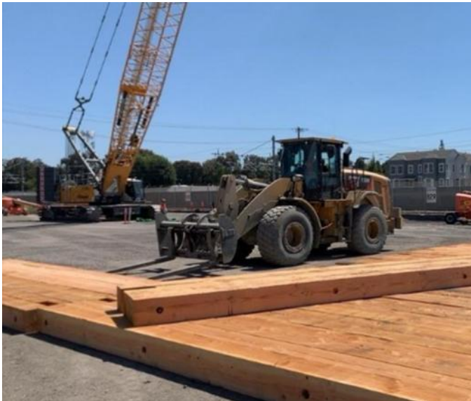
Timber matting being prepared for equipment staging and ground protection ahead of heavy lifting operations.
