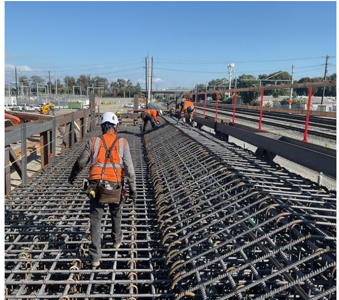
Assembly of the reinforcement cage for Y-shaped concrete panels inside the tripping frame structure.
