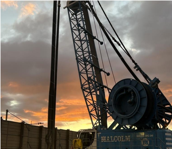
The hydromill being used to excavate materials.
