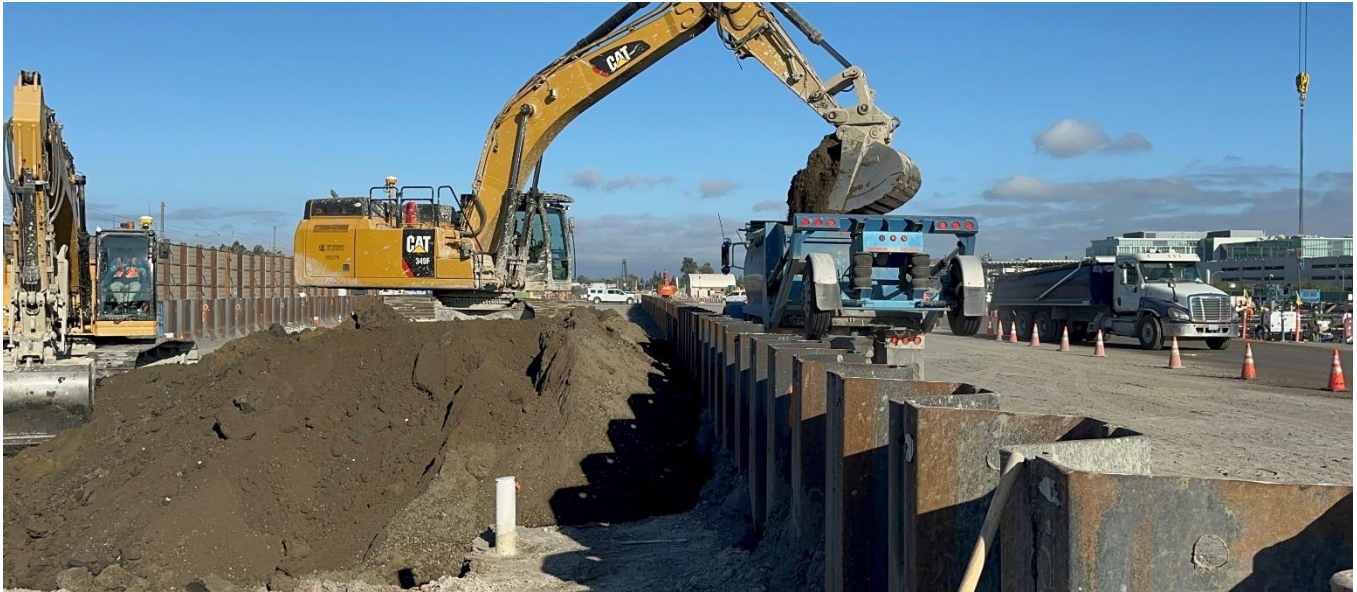
Excavation and hauling activities continue as crews remove soil to prepare for upcoming underground construction.
