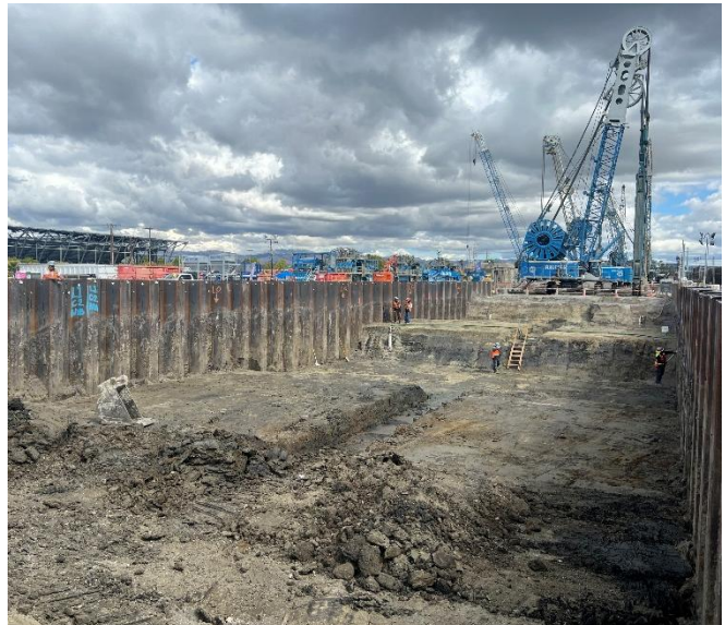
Sheet pile excavation beginning with the first cut made into the ground.
