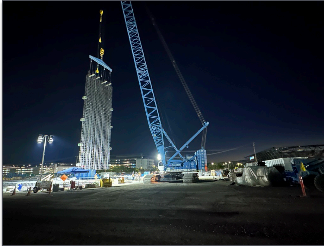
Rebar Cage Lift – Support Walls
