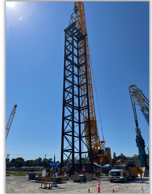
Test lift of “tripping frame”
