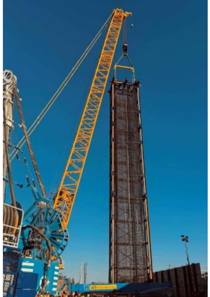
The custom-built tripping frame and LR 11000 crane allow the massive Y-panel to rotate safely and steadily into an upright position.
