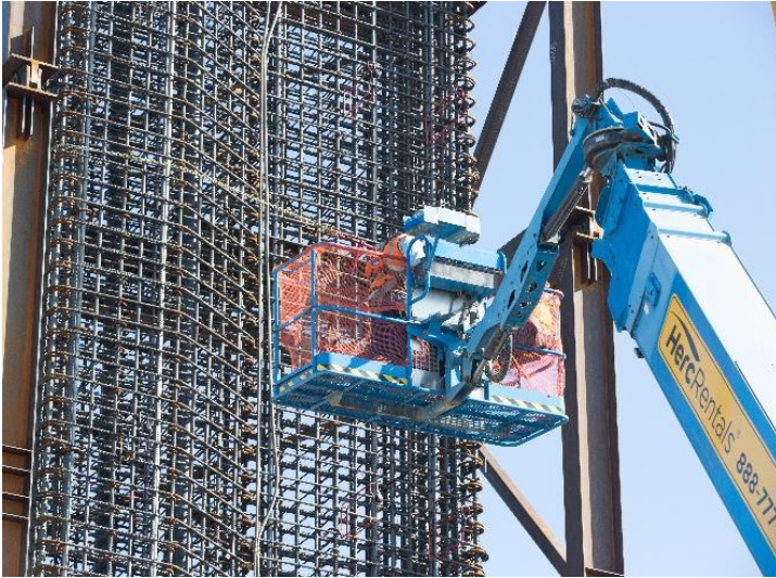
Crew members on an aerial lift inspect and guide the Y-panel rebar cage as it reaches vertical position.
