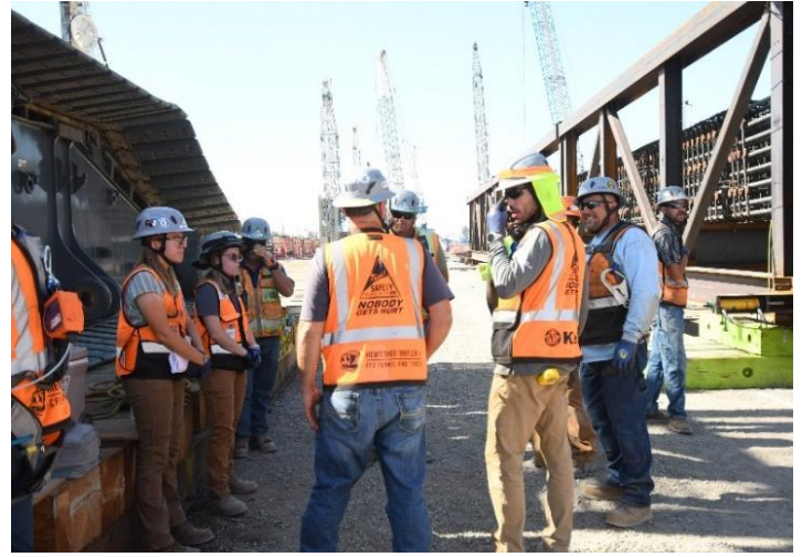
Safety is always the top priority. Crews meet regularly to plan each step of construction and keep the site safe for workers and the community.
