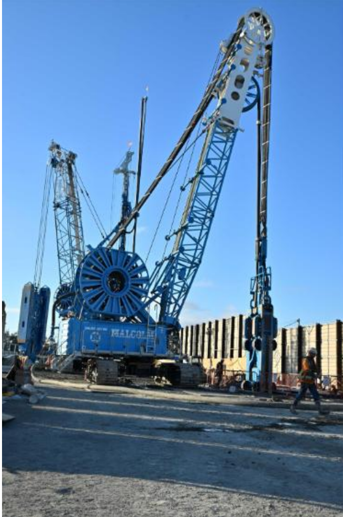
A hydromill excavates deep underground walls that will support the future tunnel and station below the surface.
