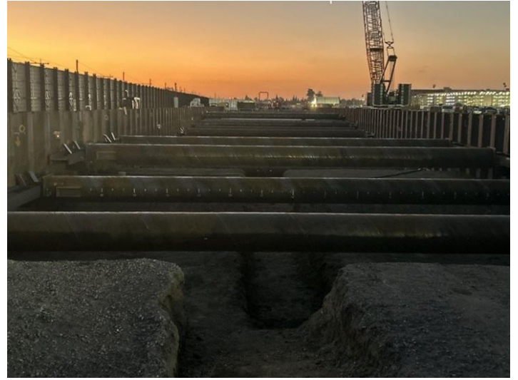
Bracing strut supports in the sheet pile wall area progresses.
