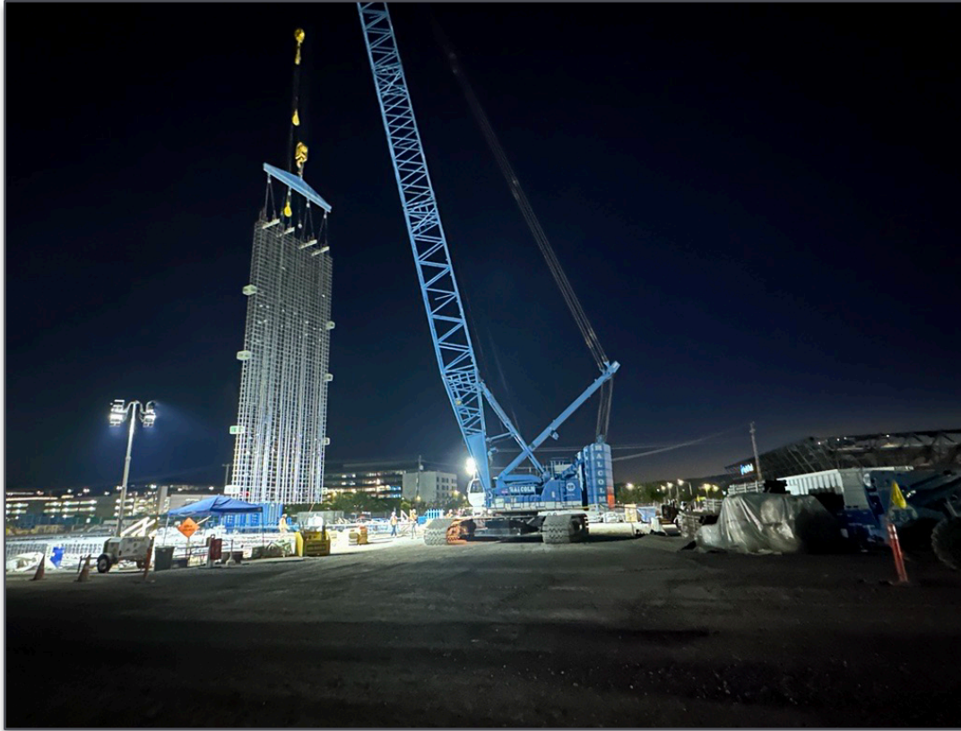
Rebar Cage Lift – Support Walls
