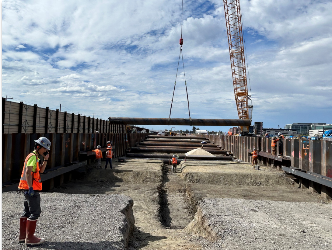
Excavation of launch structure, placement of struts and walers
