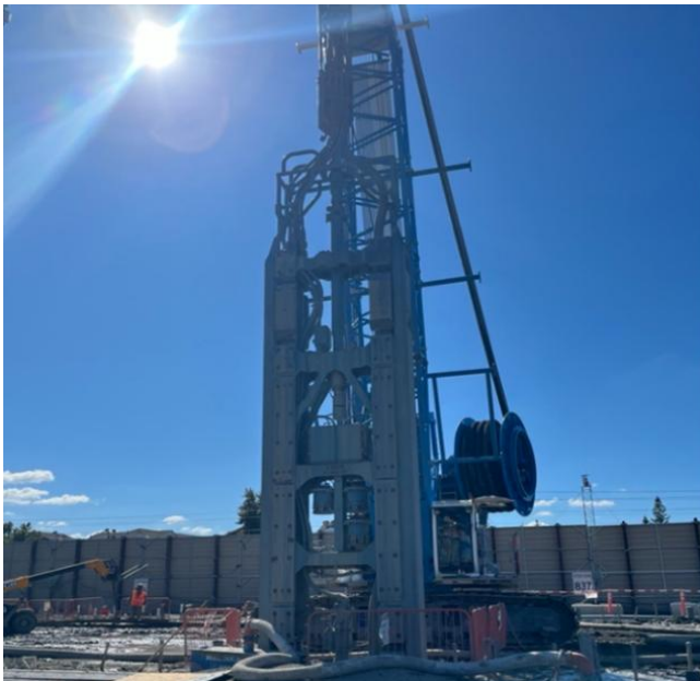
Milling a underground support wall, a reinforced concrete section that will form part of the tunnel roof, to prepare it for future construction phases.
