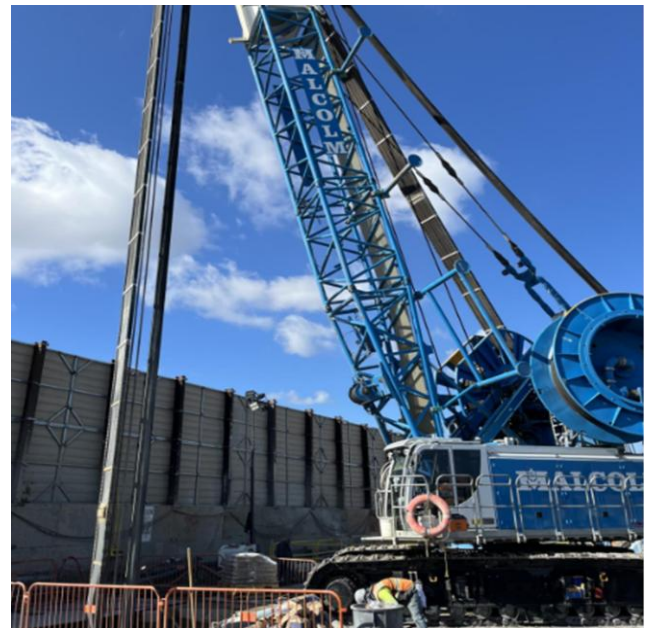
A hydromill digging machine working above a Y-Panel that has been lowered into place as part of the underground support structure.
