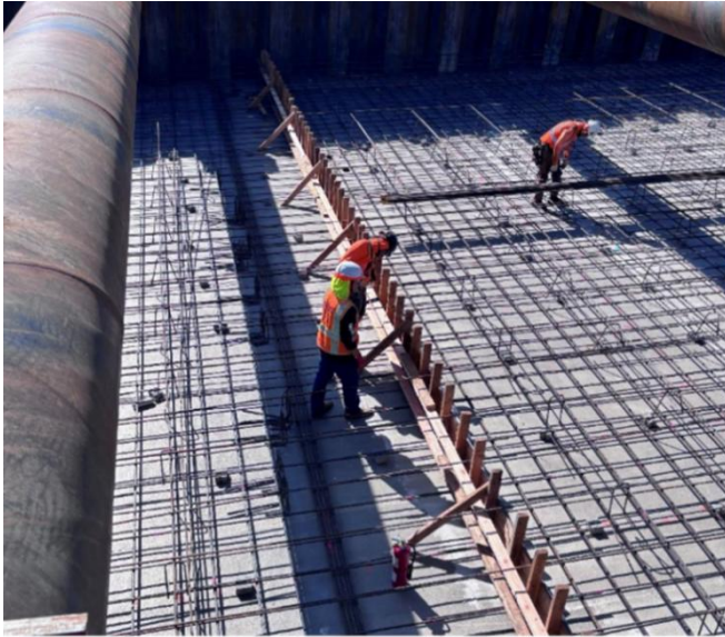
Forming a bulkhead, a temporary concrete barrier used to shape and contain the slab pour, within the sheet pile area.
