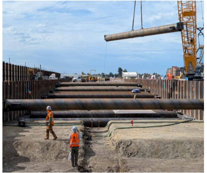
Lifting and placing steel struts onto walers, which act as horizontal braces to support the excavation walls and maintain stability during construction.
