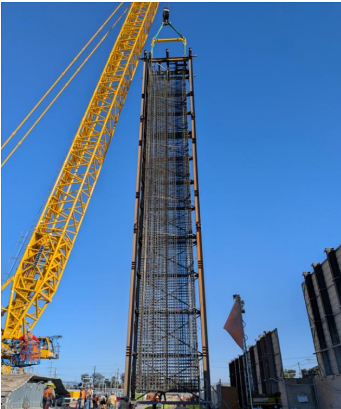
Tripping a frame, or rotating it upright, to install a Y-Panel — one of the large, reinforced concrete walls that form part of the underground structure.
