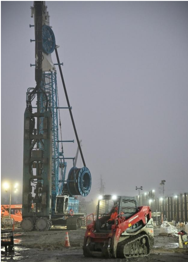
Hydraulic mill used to excavate and profile underground support walls, with a skid steer staging materials nearby.
