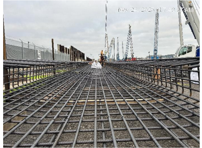
Continuing to progress rebar cage assembly at the Caterpillar Shaft.
