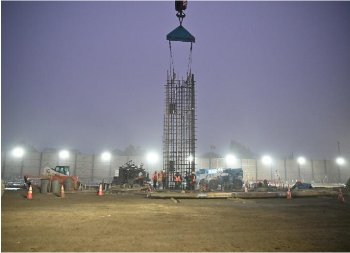
Lowering a rebar cage into the excavated hole at dawn.
