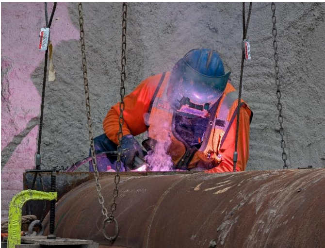
Welding of the bracing to allow the excavation to continue deeper.
