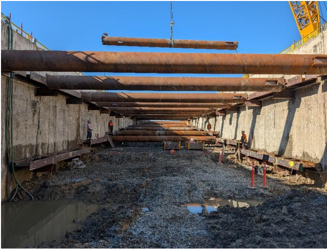
Bracing is a temporary steel support installed to stabilize the excavated support walls during construction. In this photo, we see bracing lowered into place to support the work area.
