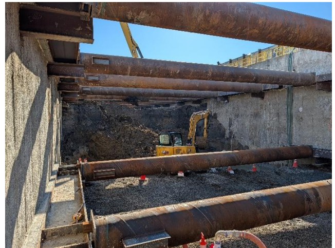
Excavation of the Launch Structure at areas where bracing struts are installed.
