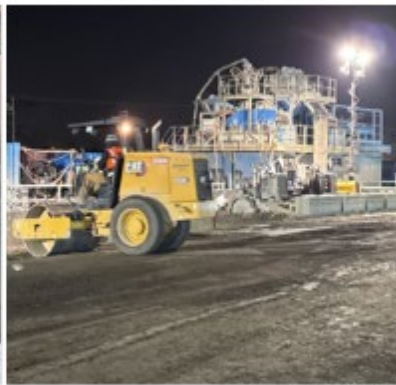
Grading and Compacting Project Site Access Road
