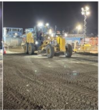
Grading and Compacting Project Site Access Road
