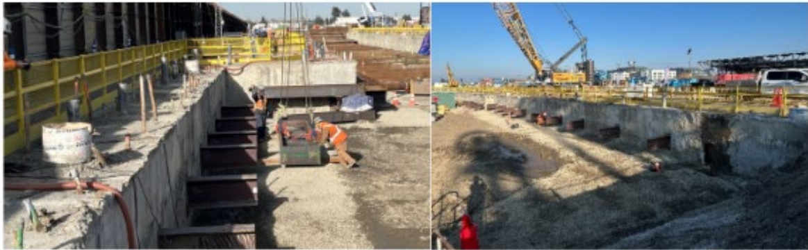
Installation of Bracing Walers in the Cut and Cover D-Wall Section
