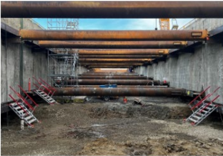
West Portal Level 2 Excavation and Bracing Overview - Looking North
