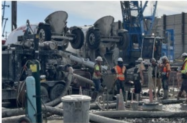
Concrete Placement of Cat Shaft Panel
