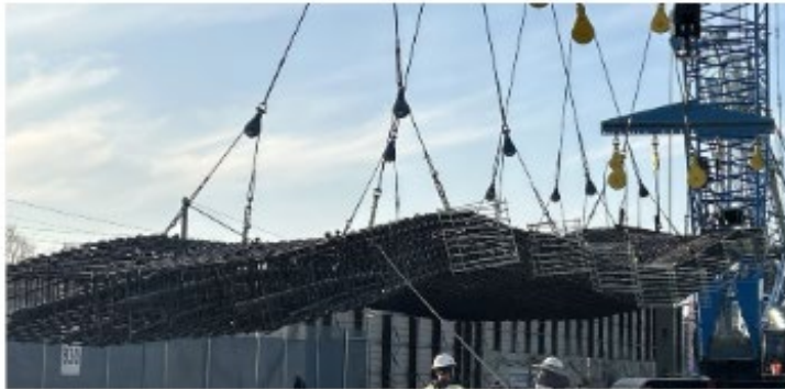
Cat-Shaft Rebar Cage Lifting Operations
