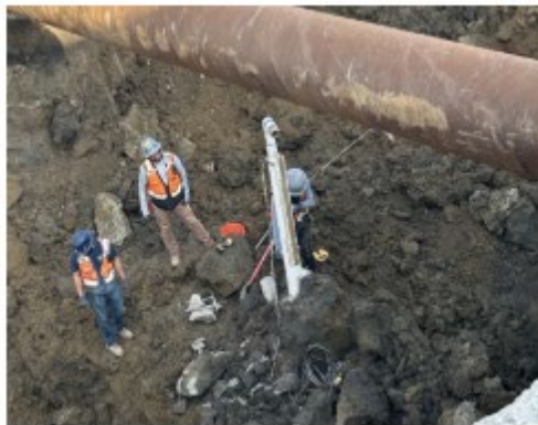
Lowering of Dewatering Wells in the Excavation Zone
