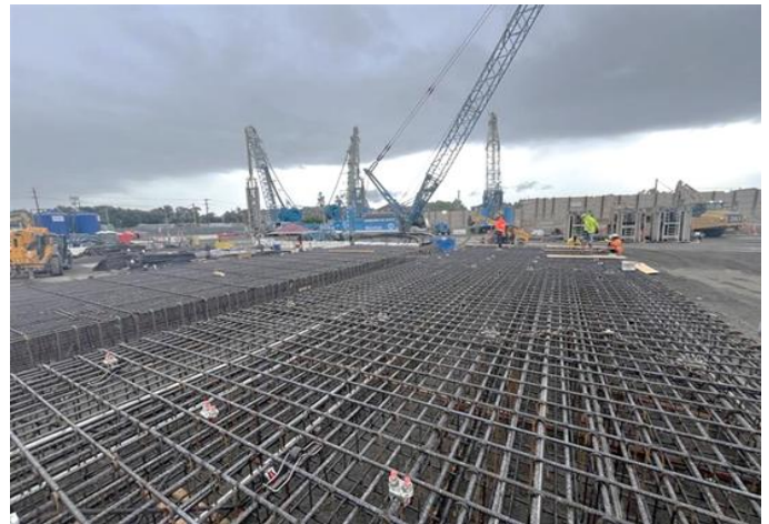
Rebar assembly for walls at front of launch structure
