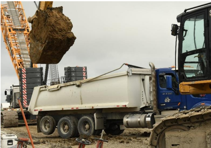
Loading excavated material into dump trucks
