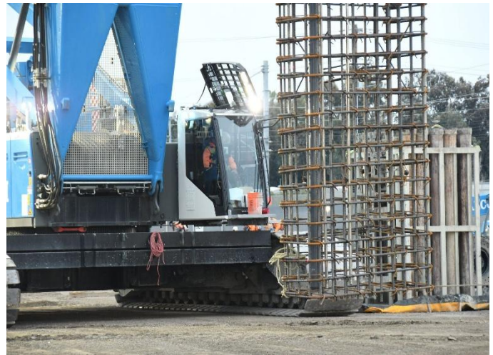
Crane operators move rebar cages to position
