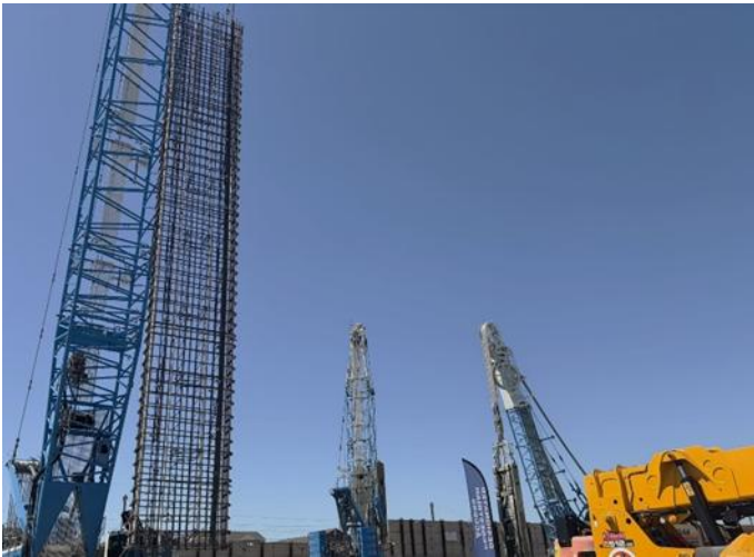
Picked rebar cage ready to be inserted into the ground
