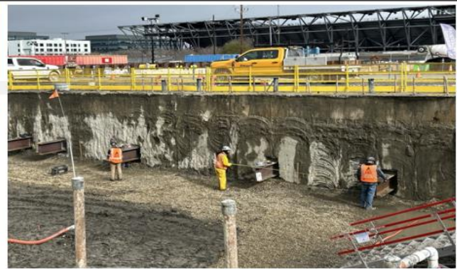
Cut & Cover Level 1 - Installation of Bracing Lookouts
