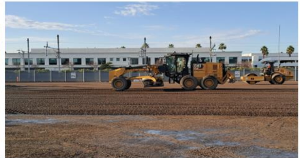
Grading and Compacting of Project Site
