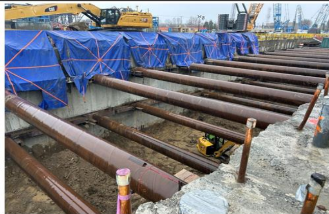
U-Wall Level 3 Mass Excavation Overview
