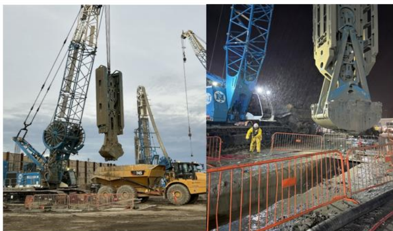
Cat Shaft Excavation using Hydraulic Grab (Day & Night Shifts)
