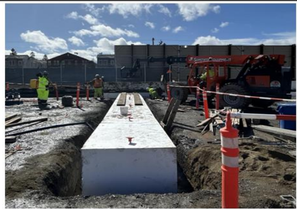
Confinement Wall Guidewall Construction
