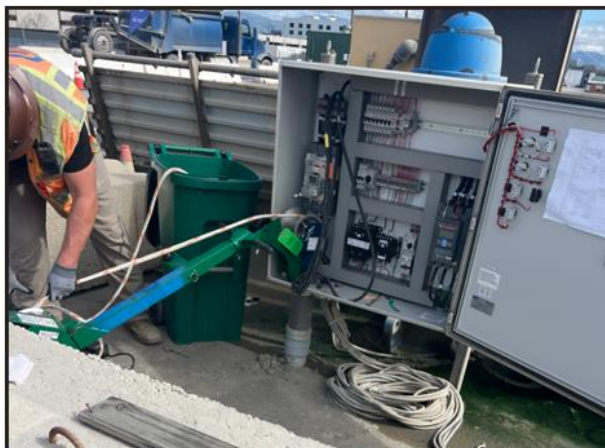
Wire Pull at Wheel Wash Station
