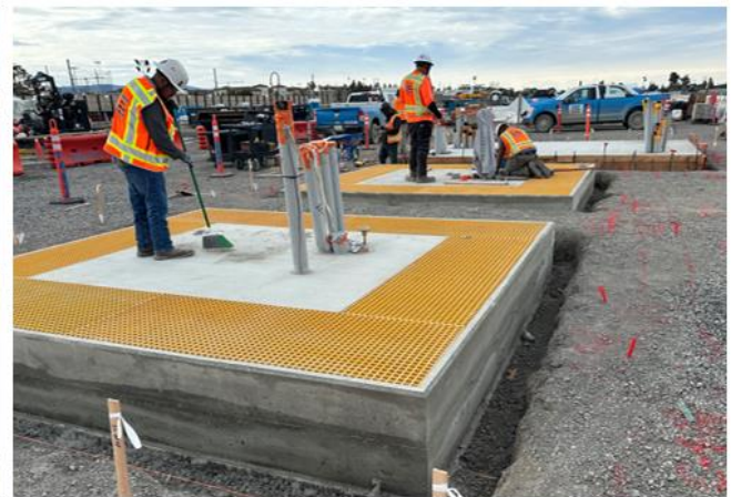
Cleaning and Conduit Cutting at Power Drop #3
