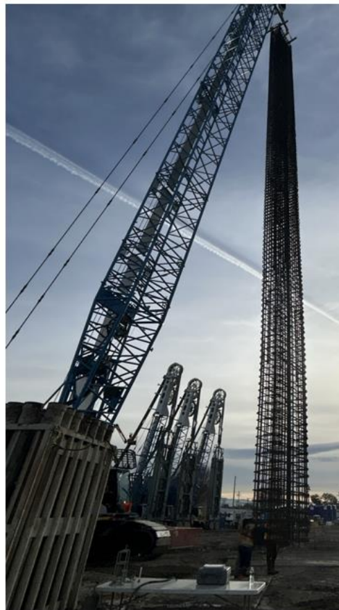
Cat Shaft Wall Rebar Cage Placement
