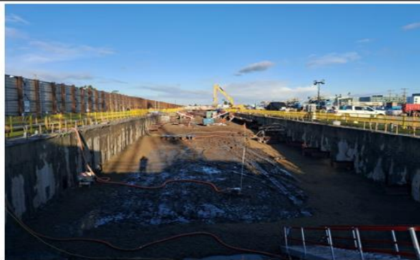
Cut & Cover Level 1 Mass Excavation Overview - Looking North
