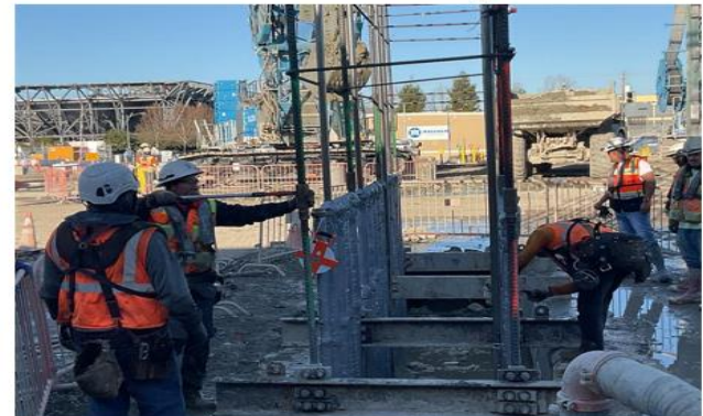
Splicing of Cat Shaft Wall Rebar Cage
