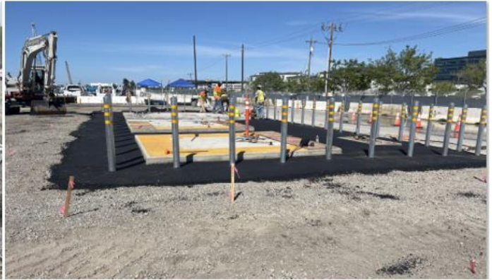
Placement of Asphalt Concrete at Power Drop #3
