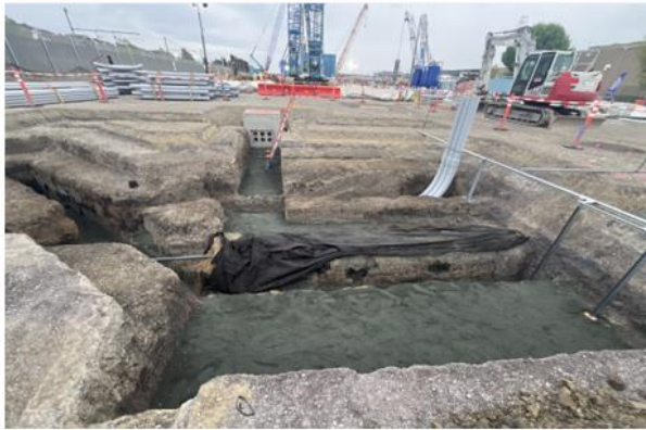
Excavation for Conduit Installation at Medium Voltage Substation (MVSS)
