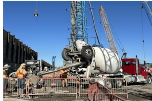
Concrete Placement of Cat Shaft Tunnel Eye Panel
