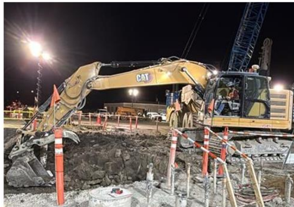
Ongoing Mass Excavation of the TBM Launch Structure
