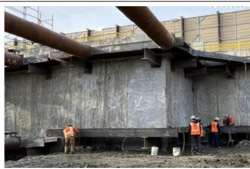
Installation of Bracing Walers on Cut & Cover D-Wall
