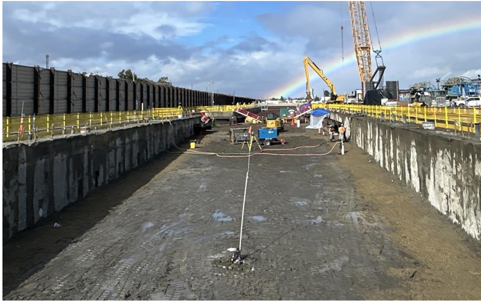
Cut and Cover Level 1 Excavation
