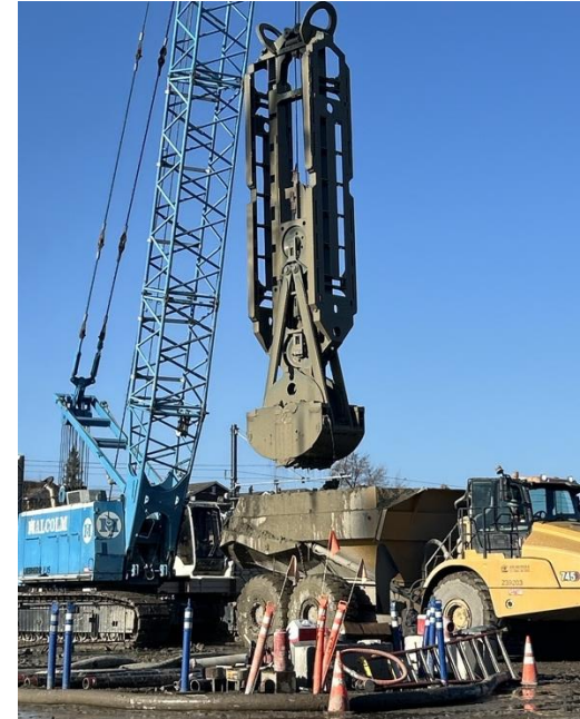
Excavation Utilizing Mechanical Grab
