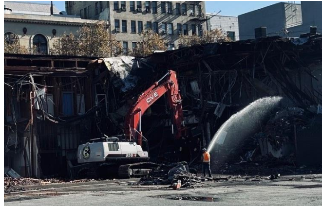
Image: Water Hose in use during demo of building downtown
