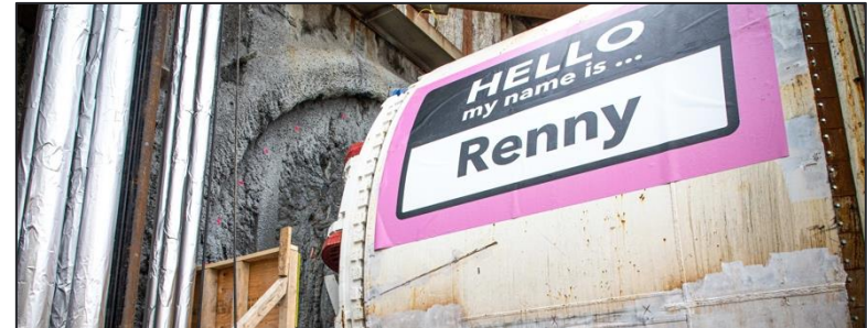
Eglinton Crosstown West Extension
