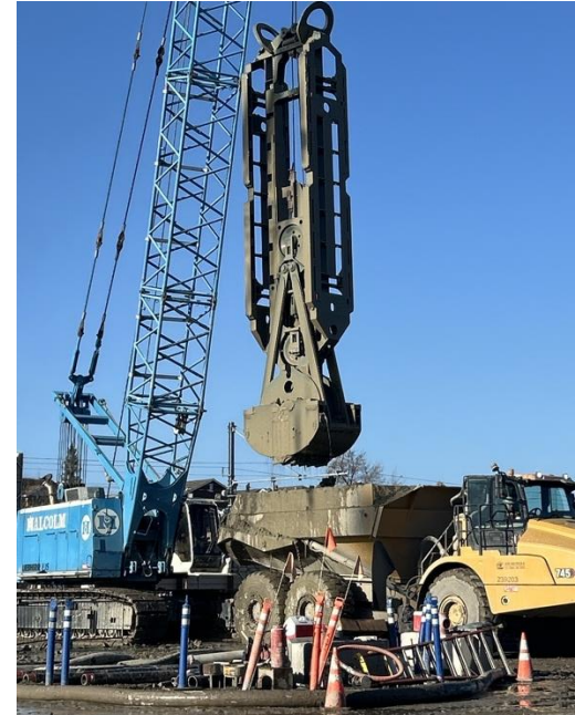
Excavation Utilizing Mechanical Grab
