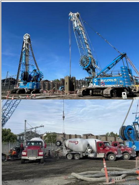
Excavation and Concrete Placement of Confinement Wall Panels
