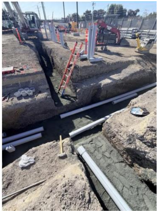
Installation & Trenching of Conduits & Underground Infrastructure at the MVSS
