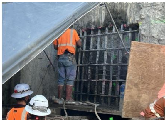
Repairs of Cut & Cover D-Wall Panel P26
