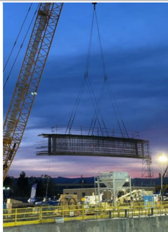
Lifting Cap Beam Top Strut Rebar Cage
