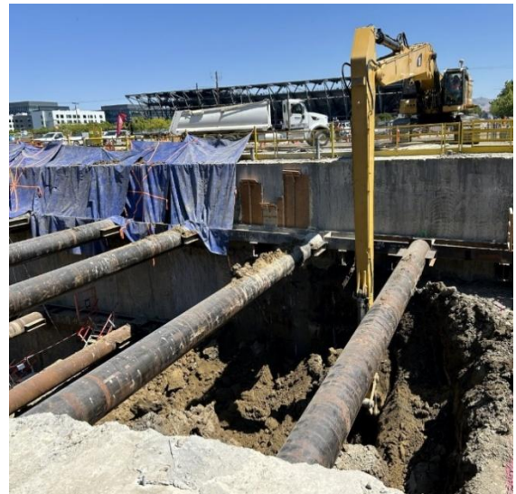
Long Reach Excavator between Level 1 and 2
