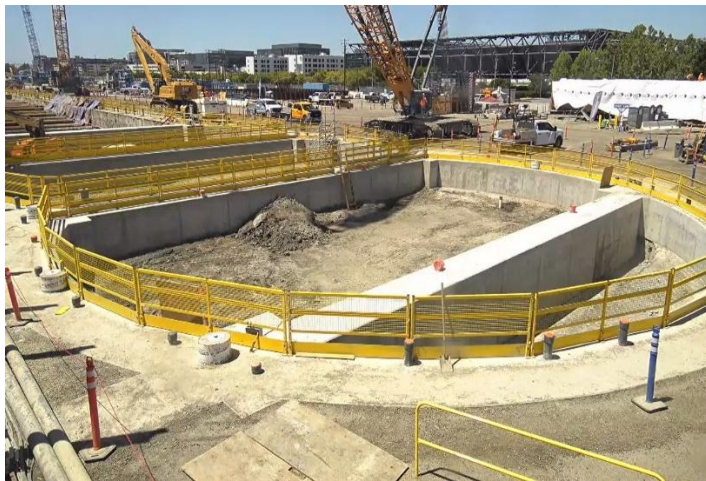
Caterpillar Shaft Completion Overview and Handrail
