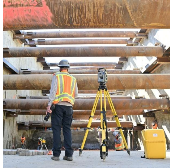
Survey crews scanning the launch structure as excavation and strut installation progresses
