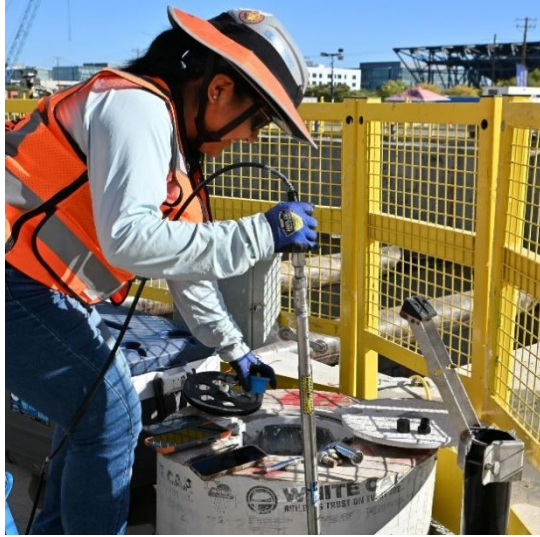
Crew member installing inclinometers
