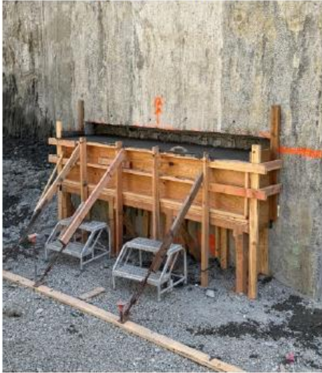
CAT Shaft - Level 1 Bracing Supports Formwork
