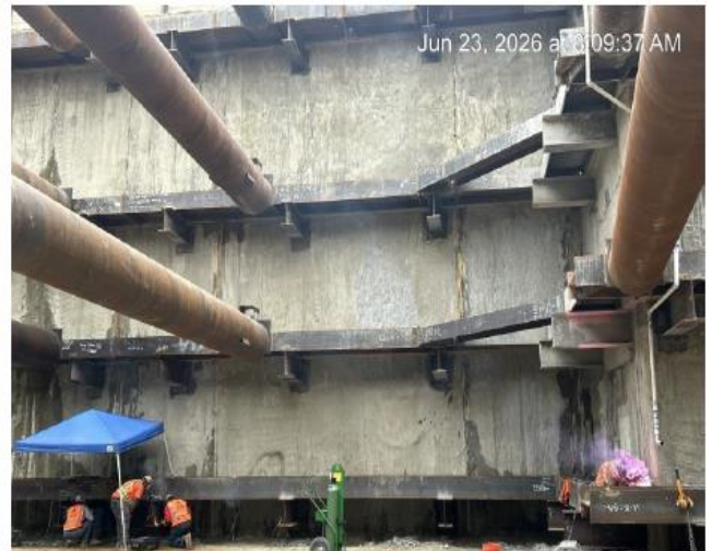
Cut & Cover – Level 4 Bracing Installation
