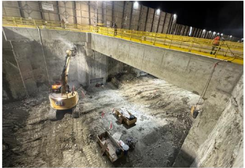
CAT Shaft – Grinding of D-Walls
