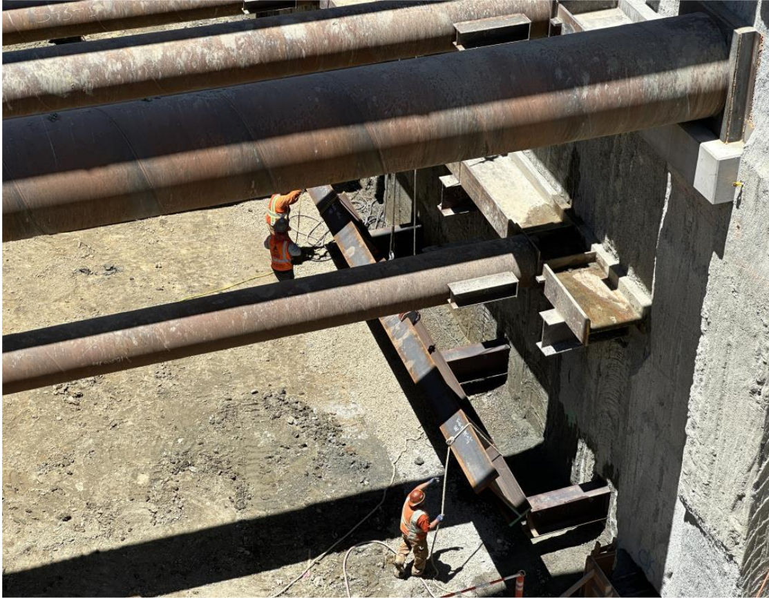
Cut and Cover – Water Installation
