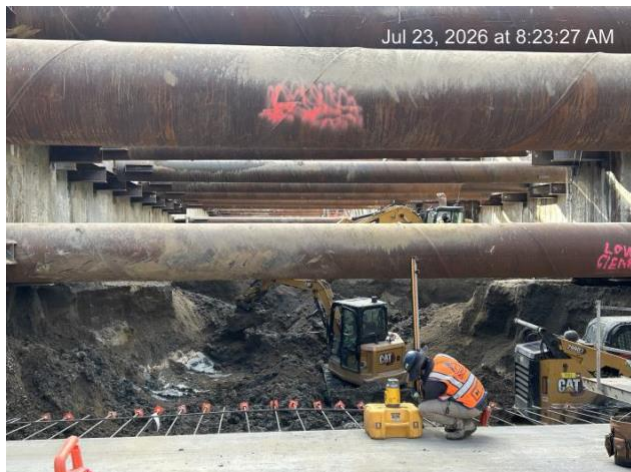
Cut and Cover – Subgrade excavation
