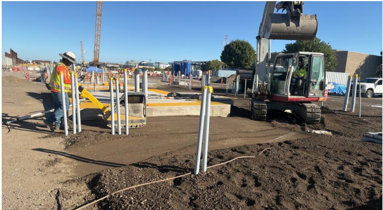
MVSS – Ground Grid back fill and compaction
