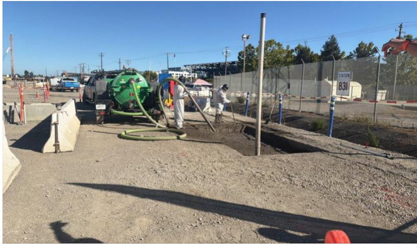
Transformer Pad T3A excavation
