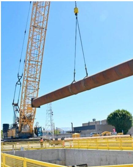
Crane lowering temporary support beam into Launch Structure.
