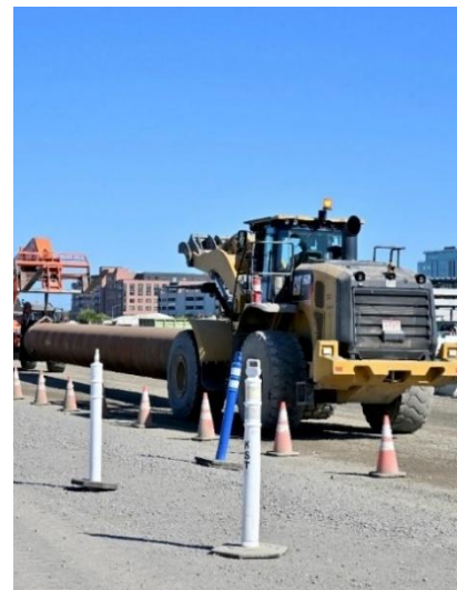
Heavy loader transporting a steel strut.
