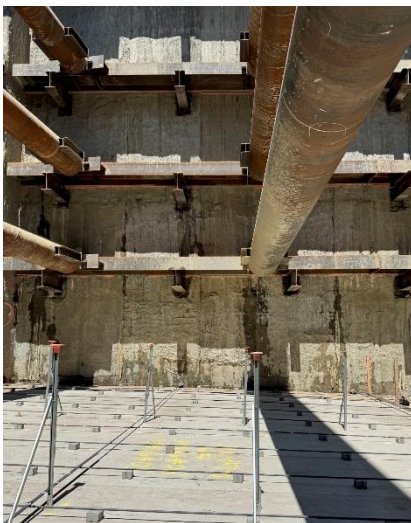
Rebar and formwork in place before concrete pour for working slab.
