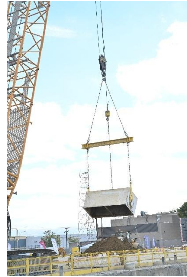
One of the last buckets of excavated material to come out of the West Portal Launch Structure.
