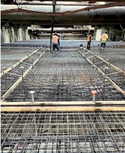
Crews installing rebar before the working slab concrete pour.
