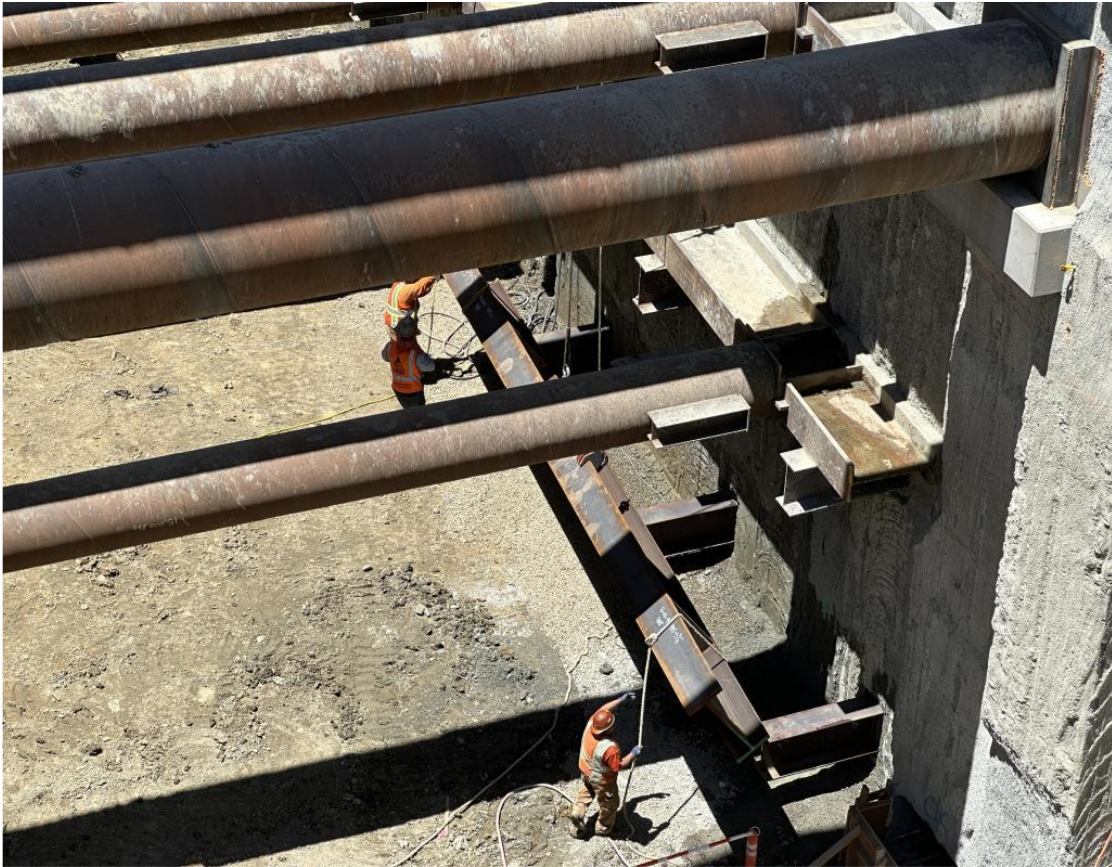
Cut and Cover – Water Installation
