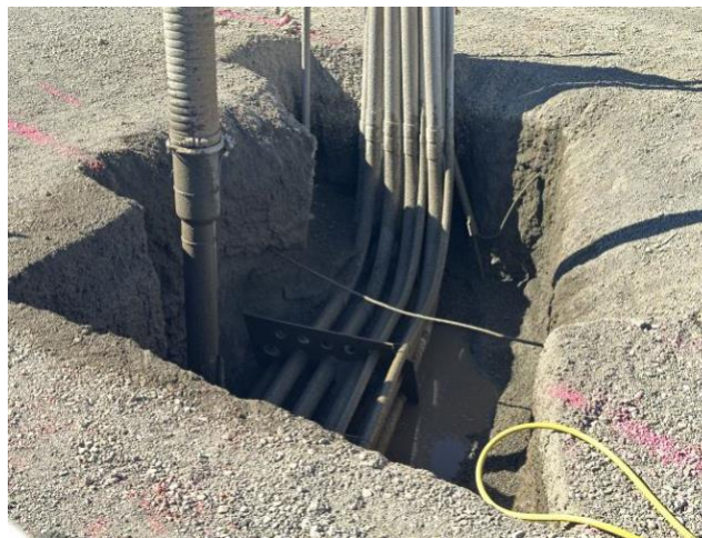
Air Compressor – Conduits exposed for relocation
