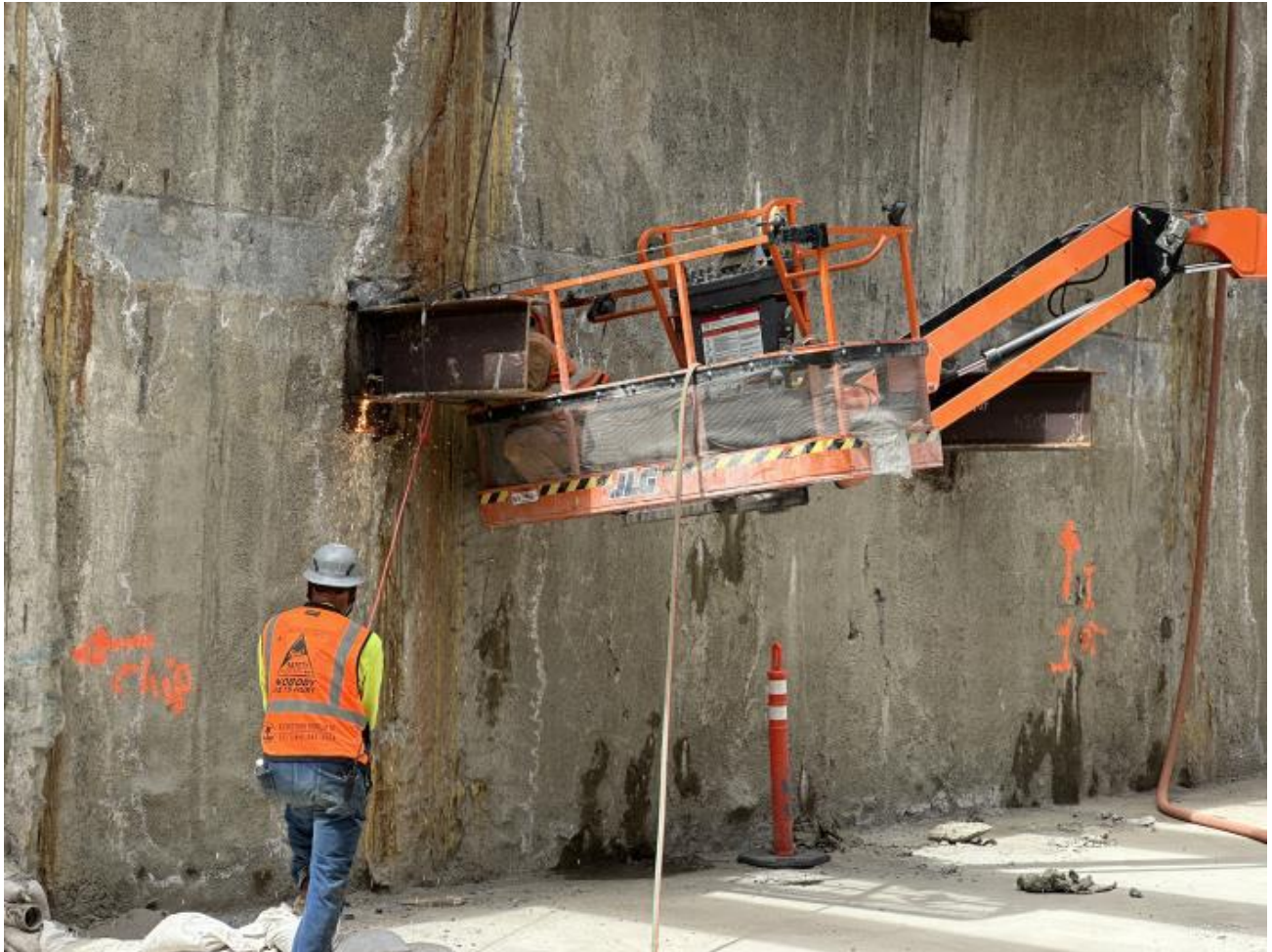
U Wall – Bracing Removal
