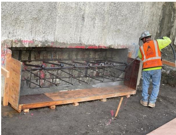
CAT Shaft – Corbel Installation
