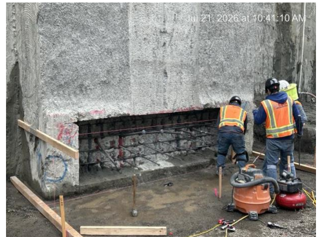
CAT Shaft – Corbel Installation
