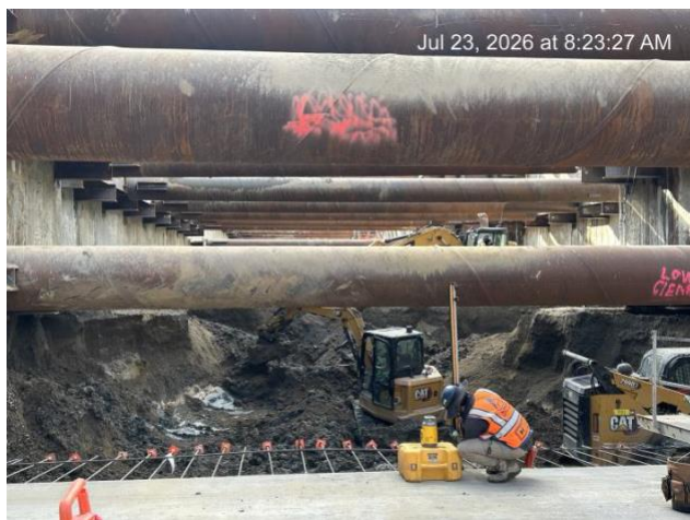
Cut and Cover – Subgrade excavation
