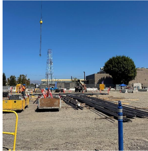
Rebar staged in preparation for concrete slab in the caterpillar shaft
