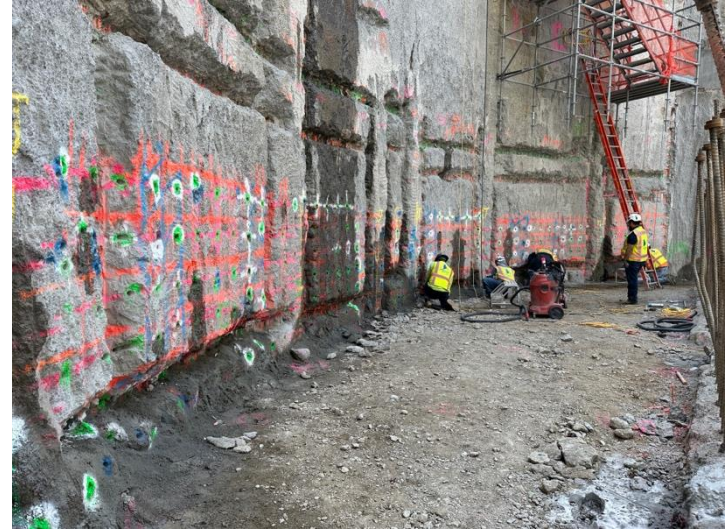
Drilling dowels from inside the Caterpillar Shaft
