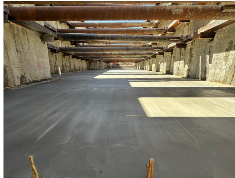
Cut and Cover Working Slab Mud Mat Complete
