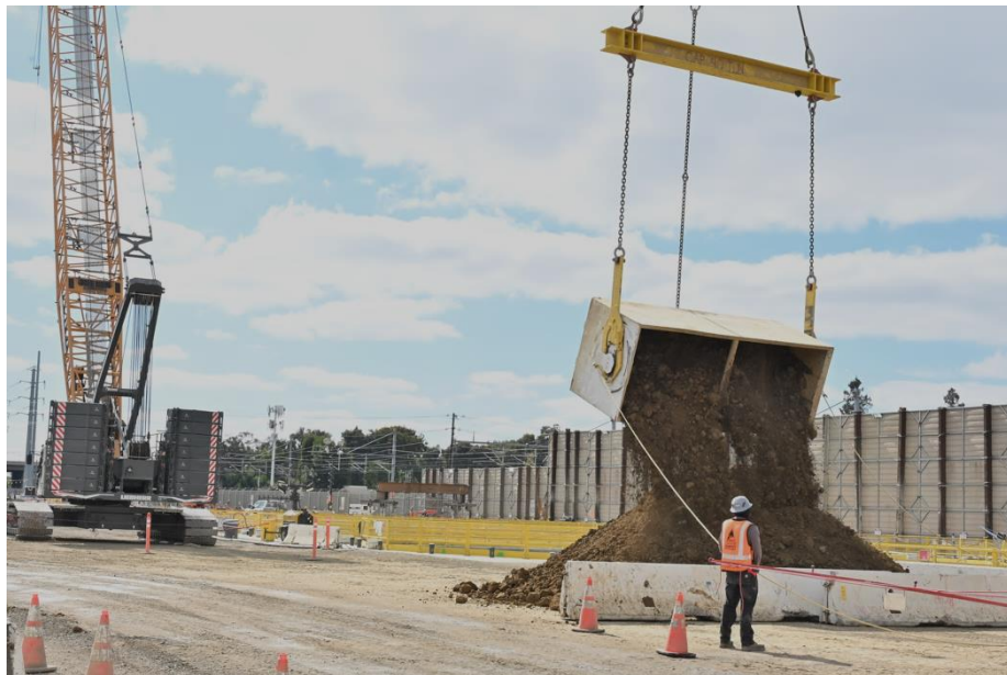
One of the last buckets of excavated material to come out of the West Portal Launch Structure
